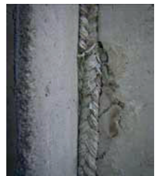
Joints de dilatation
