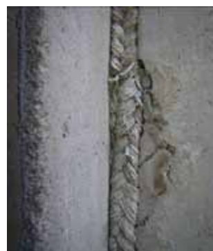
Joints de dilatation
